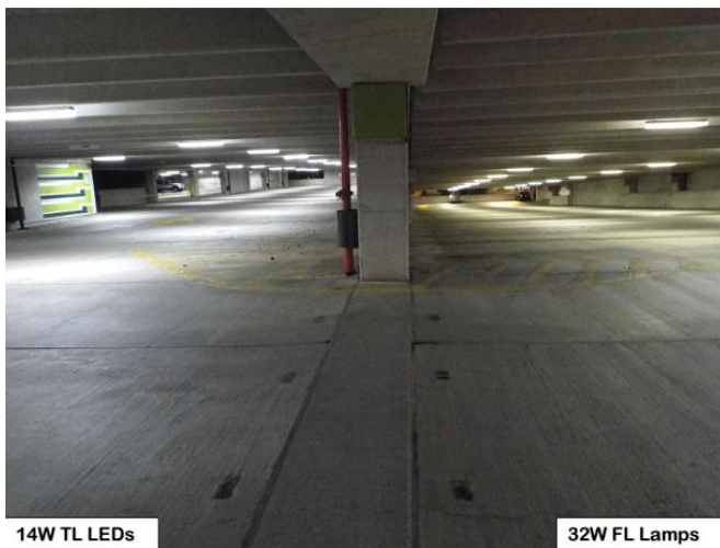
ThinkLite replaced 32W FL lamps with 14W T8 LEDs highly increasing efficiency and light levels.
