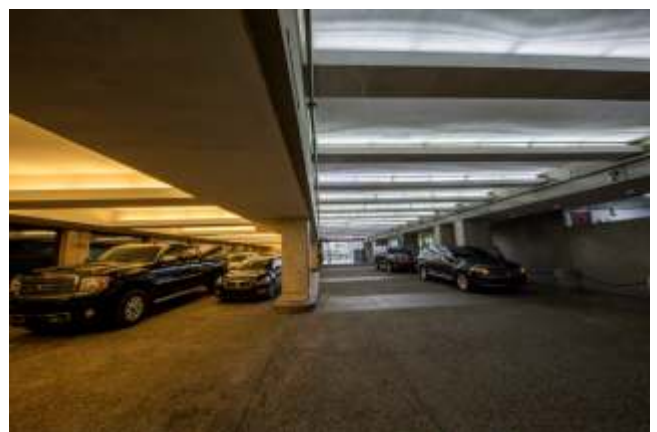
What a contrast! The adjacent hotel entrance is lit with traditional fluorescent lights while the One Post Office Square breezeway enjoys ThinkLite LED.
